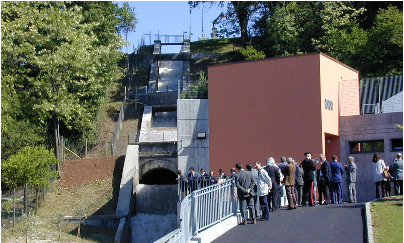
The Power Plant seen from valley
